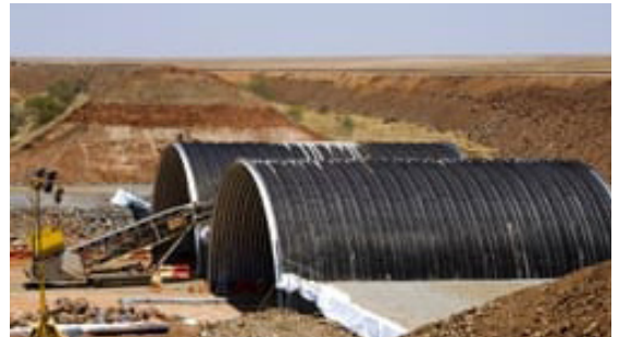
Twin Super•Cor Arches being installed.
